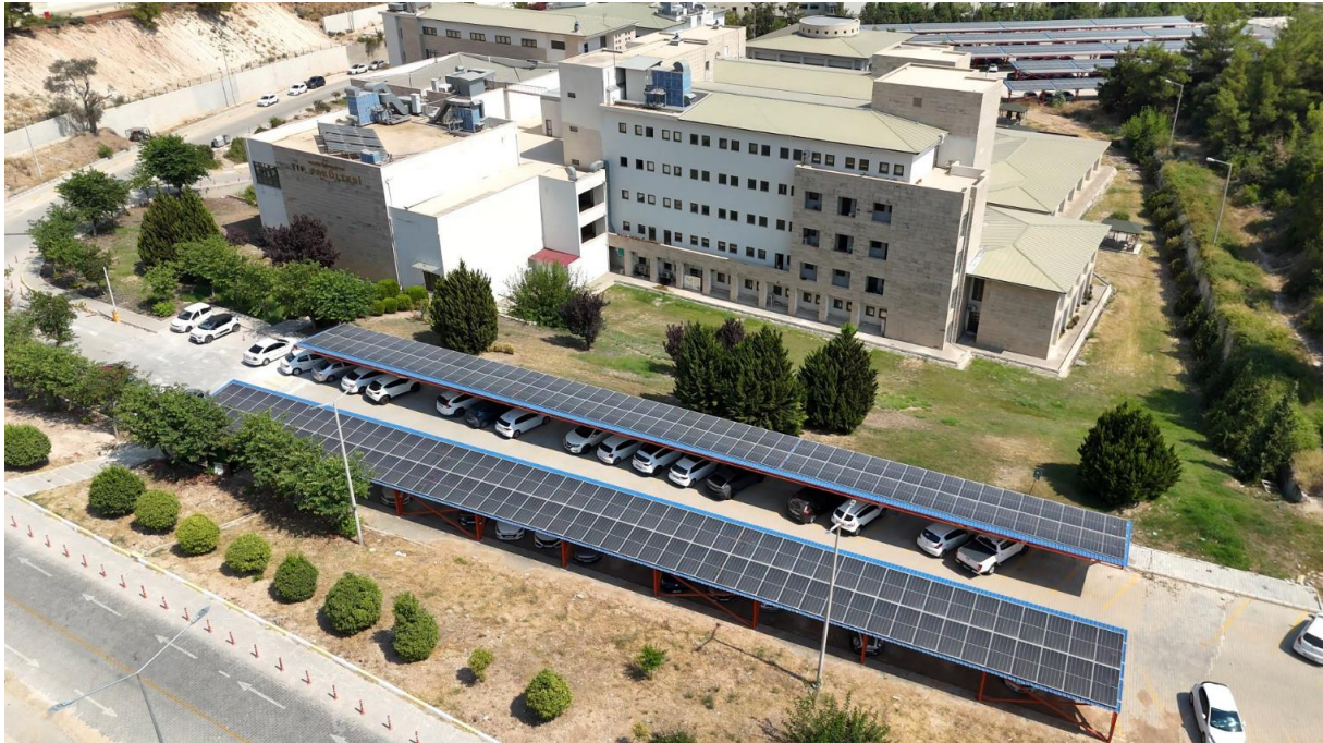
Figure 11: Solar panels constructed under KABEV Project in the Faculty of Medicine car parking area
