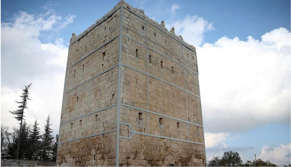
Figure 10: The restorations works on the five-storey, 30-metre-high Hellenistic Tower where the Priest-Kings resided in the ancient city of Uzuncaburç
